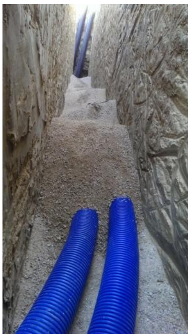
Air tubes with diameter 20cm
