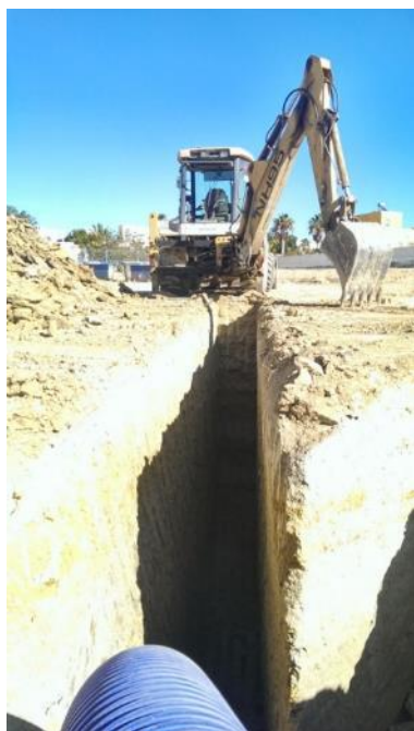
Air tubes with diameter 20cm
