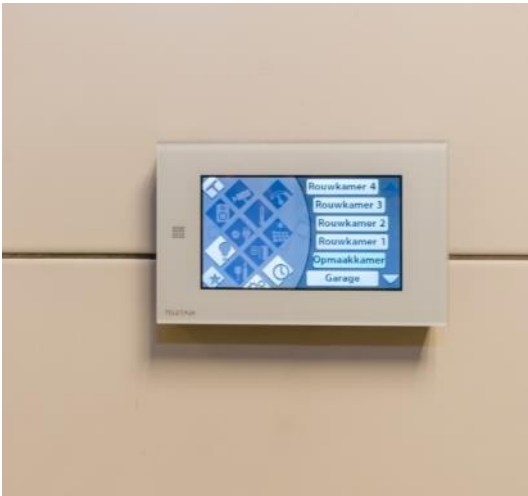
AURUS-TFT touch panels are used to manage the different rooms
