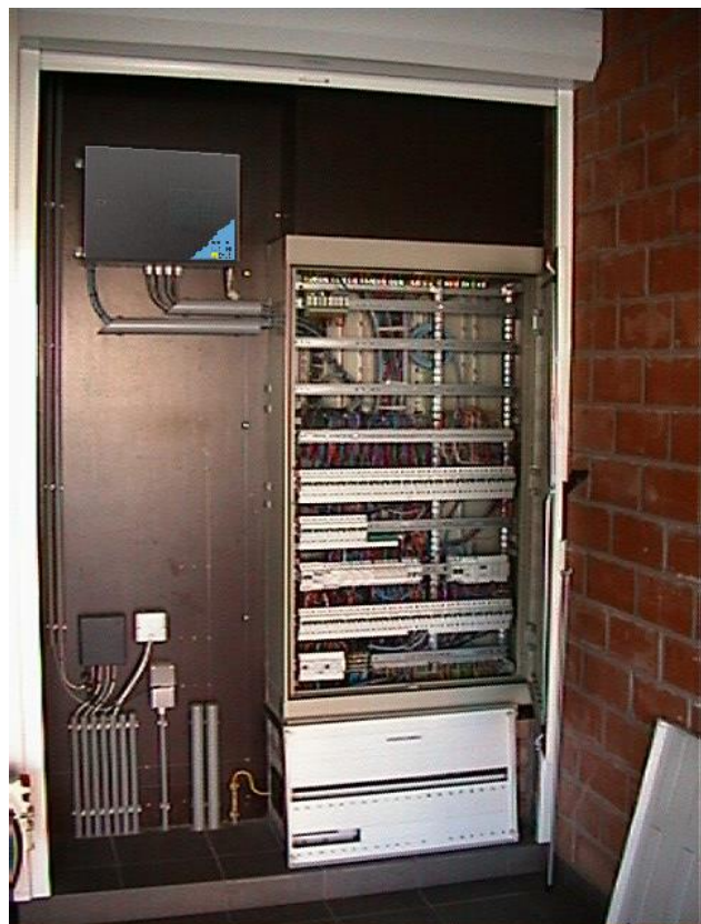
Figure 2: Clear division between input and output cables
