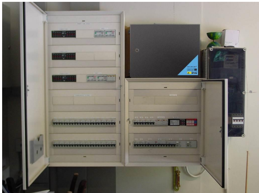
Figure 1: MICROS+ outside distribution board
